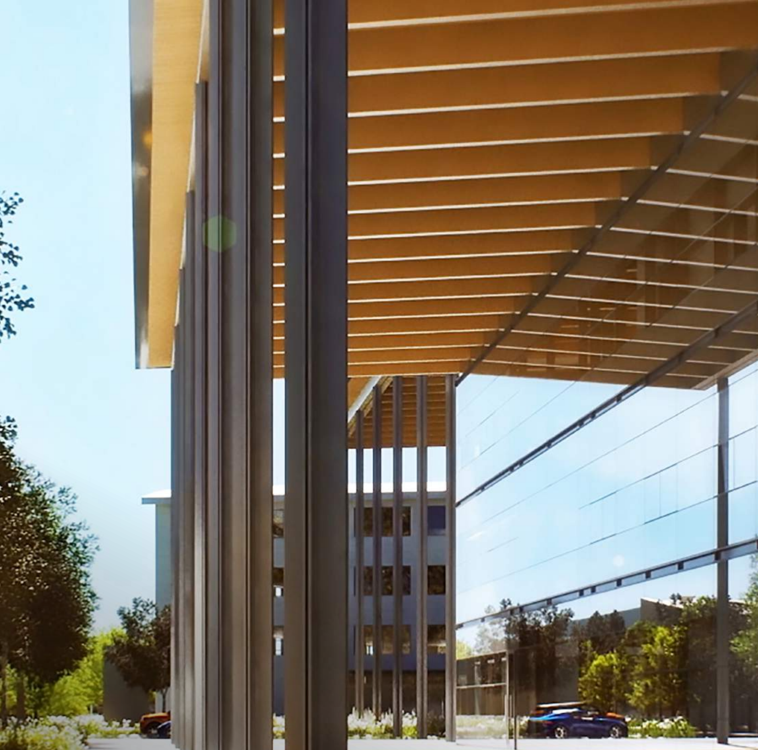
— The Design and Engineering HQ for Jaguar Land Rover features a roof made up of approximately 16,000m 2 of Cross Laminated Timber
